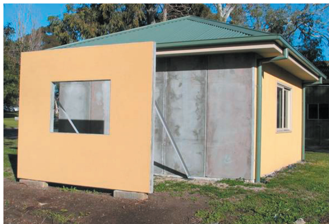
Demonstration HySSIL™ building panels at CSIRO, Highett, Victoria
